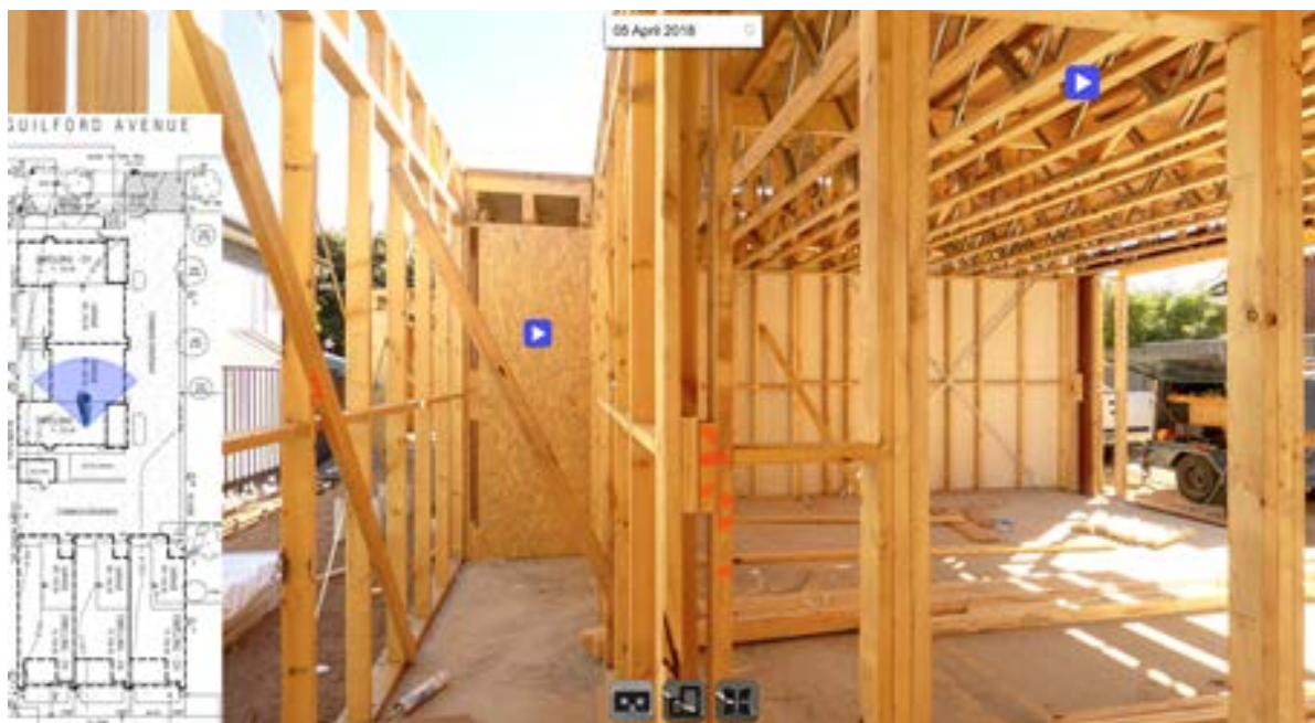
Figure 2 - Augmented 360 Panoramic Views of Timber Framing (Source: https://uo.unisa.edu.au/course/view.php?id=1322 )
