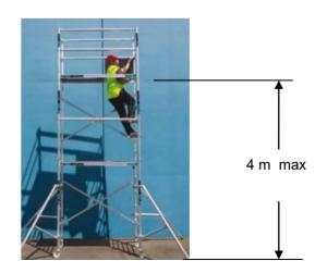
Harness & Lanyard NB. A fall arrestor requires 6.5 meter to function safety
