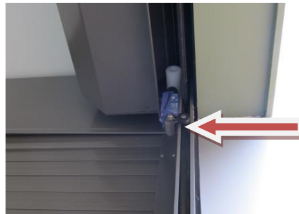
Diagram 2. Gas Shut Off Switch
